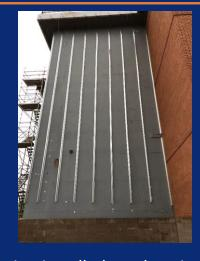
Z-girts installed on elevation D
