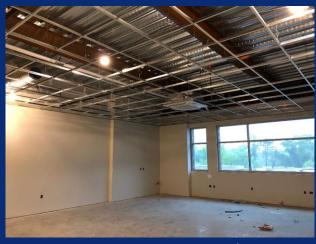
Ceiling grid installed in 2<sup>nd</sup> level classrooms
