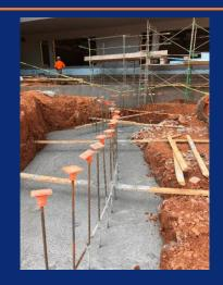
Footings poured for retaining wall B, near south stairs
