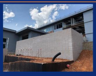
ACMU install on retaining wall F
