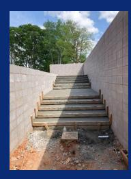
Steps poured between retaining walls E and F, near lower level entrance
